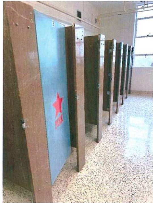
Photo A10 First Floor – Toilet partitions
