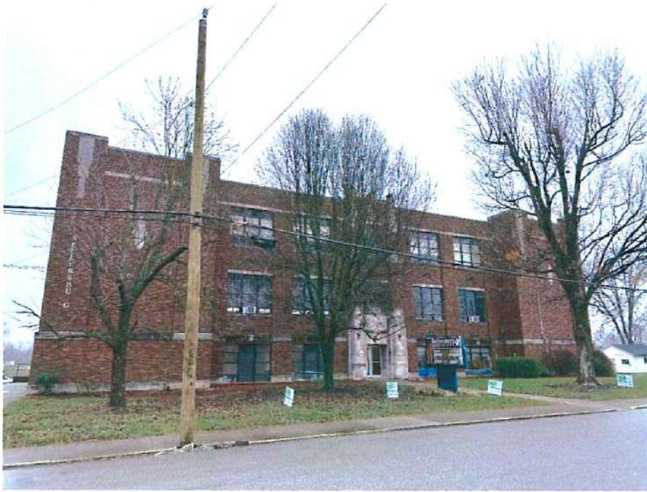
Photo A20 Exterior – West elevation
