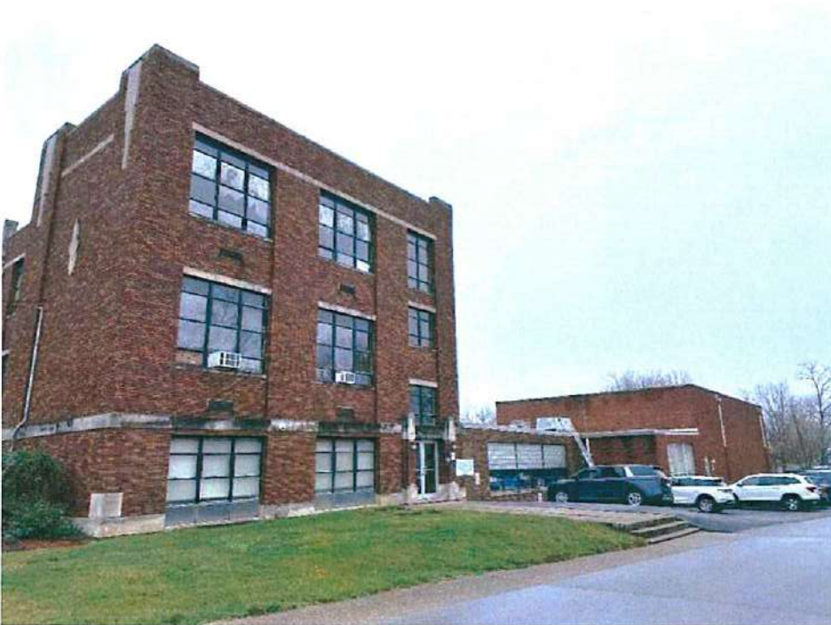
Photo A21 Exterior – South elevation
