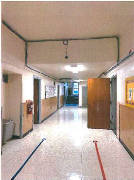
Photo A1 First Floor - Corridor
