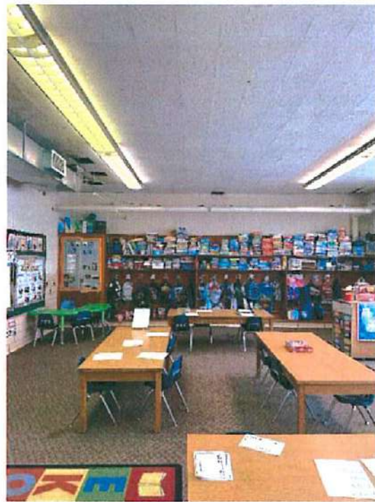
Photo A2 First Floor - Room 2; Typical conditions of first floor classroom in original section of building
