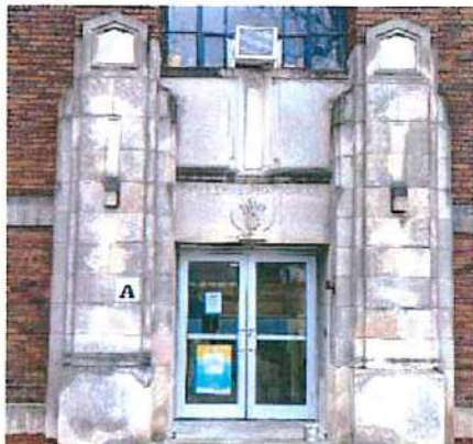
Photo E18 Existing Lighting – Exterior Metal Halide
