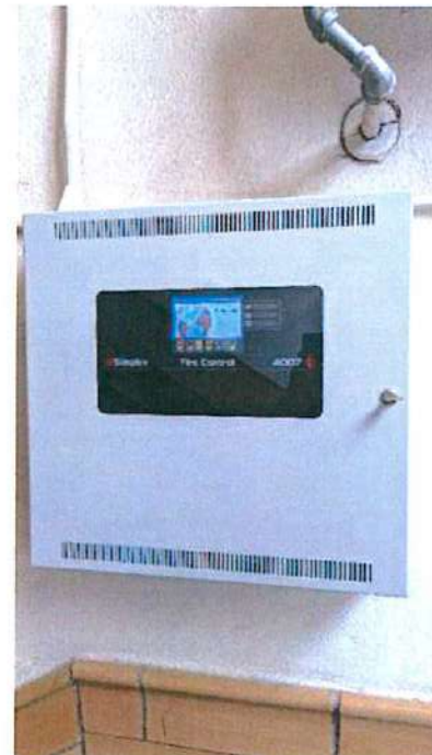
Photo E8 New FACP – 1 st Fl Plan West Entry
