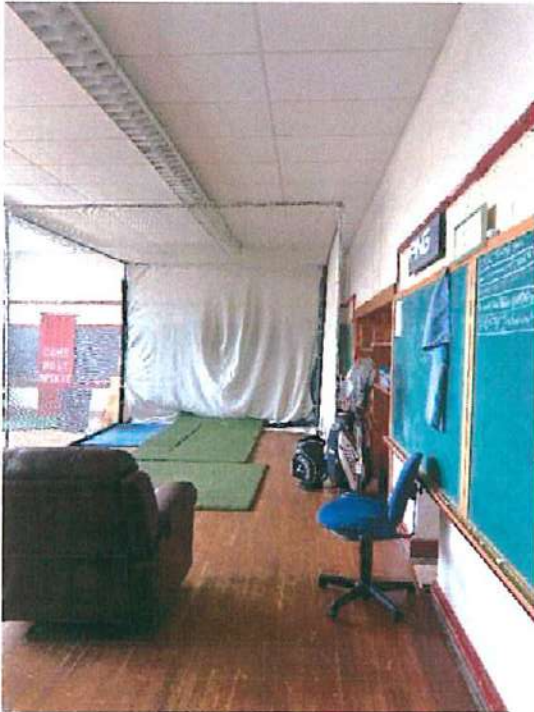
Photo A13 Third Floor – Wood flooring in classrooms
