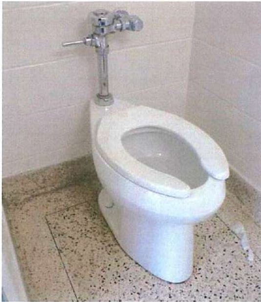
Photo M/P21 Typical Water Closet
