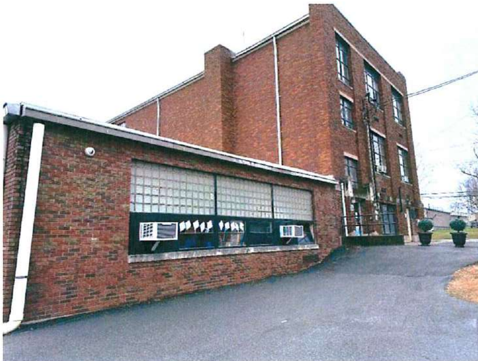
Photo A23 Exterior – Partial north elevation
