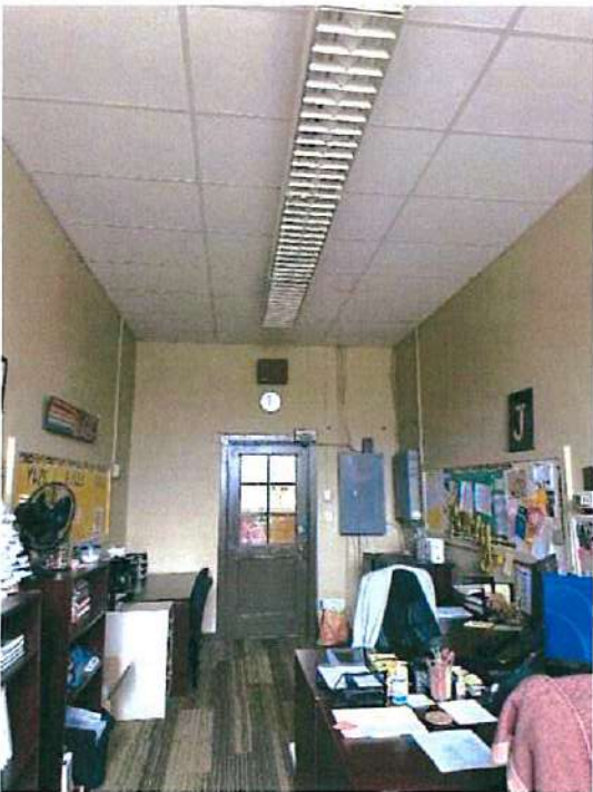
Photo A11 Second Floor – Office
