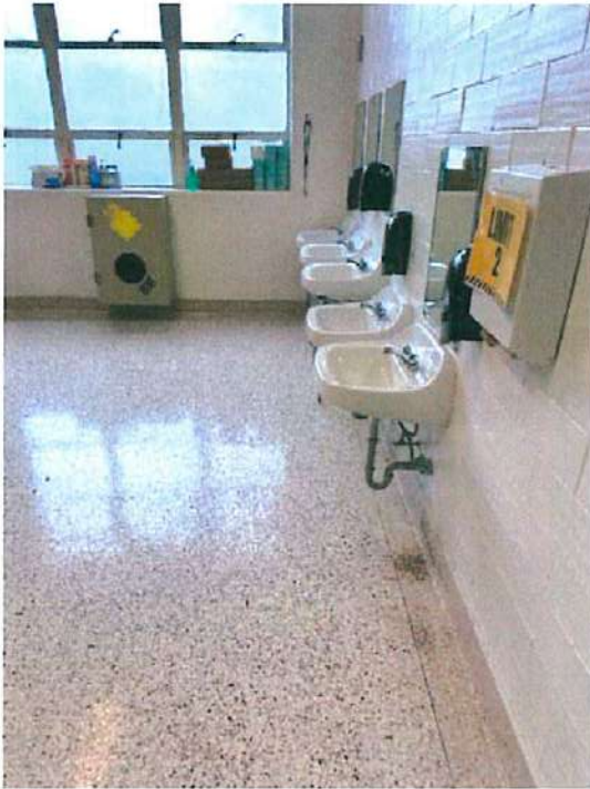
Photo A9 First Floor – Restroom sinks that will need to be adjusted in height for adults.
