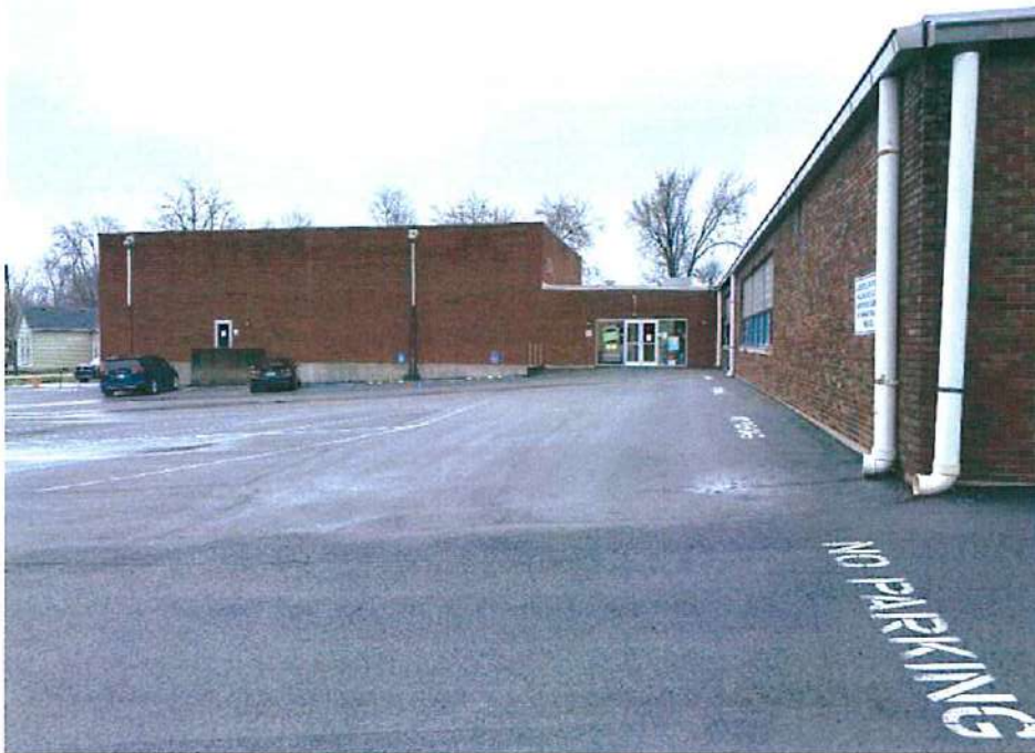
Photo A22 Exterior – Partial north elevation
